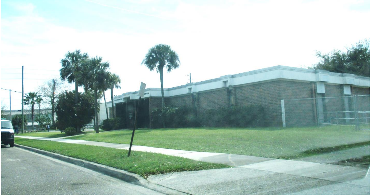
Property to the South: Butledge H. Pearson Service Center Source: Planning & Development Department 03/11/2019
